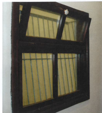
Figure 2. There should be a wire mesh or iron bars covering glass in stables to prevent horses from injuring themselves.
