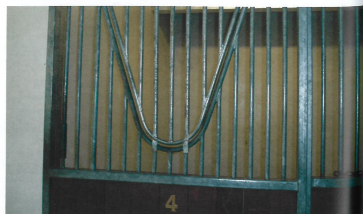
Figure 6. Door grills are used to prevent the horse from being able to get its head over the stable door and damage indwelling intravenous catheters.
