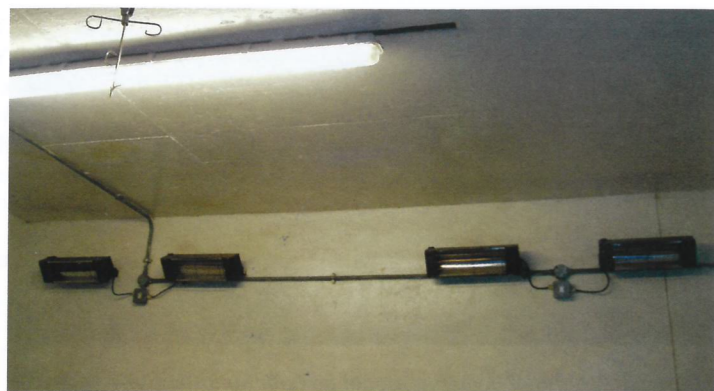
Figure 4. Permanent heat lamps are a good source of supplementary heat for sick horses.
