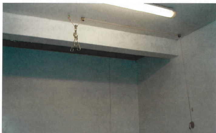
Figure 5. Fluid hangers are hooks attached to the ceiling used for suspending intravenous fluid bags.
