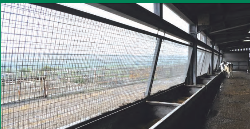
Although some of the troughs are on the outside of the building, the mesh screens have been designed to swing in, to allow feed to be deposited before they are fastened back again.
