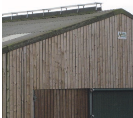
Cap protecting the 30cm open ridge, but not reducing the available outlet area, by sitting 15cm above it.
