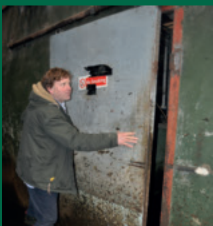
Concentrates are fed in the parlour. To prevent badgers entering, a sliding door and roller door have been installed at either end, and these are kept shut at night
